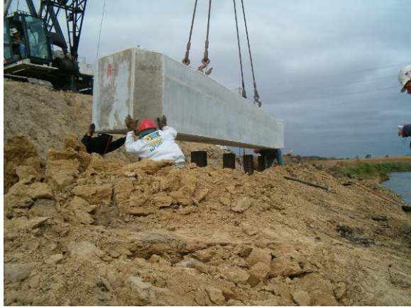
Figure 5. Setting precast abutment
