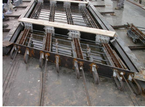
Figure 4. Longitudinal joint reinforcing
