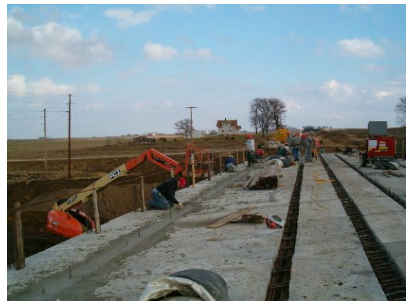
Figure 10. Casting longitudinal joints
