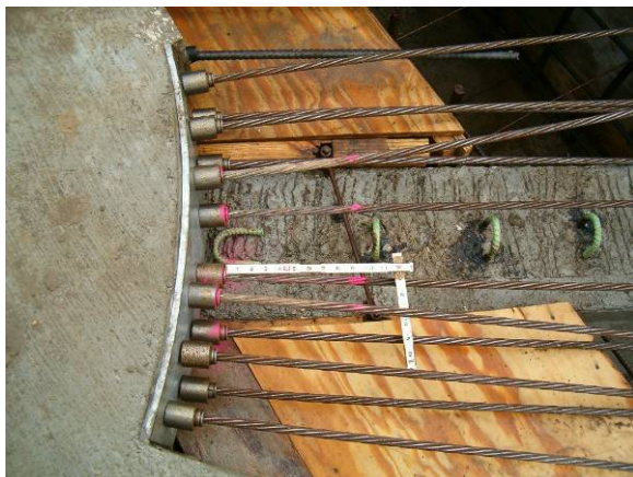
Figure 9. Strand elongation check
