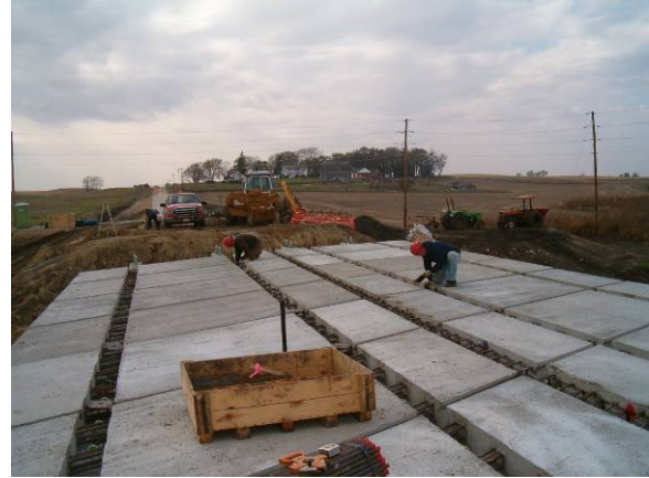
Figure 8. Leveling device installation
