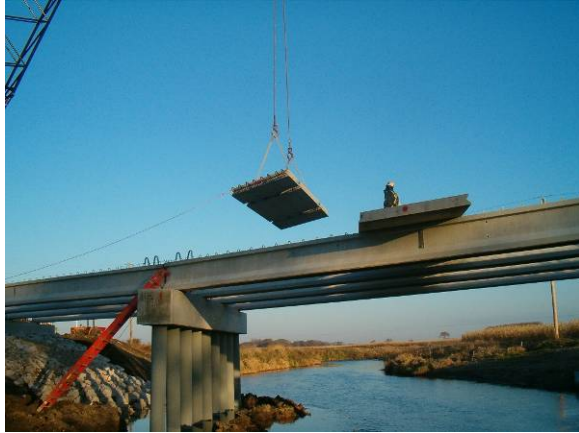
Figure 7. Deck panel erection
