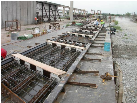
Figure 1. Panel forms and reinforcing
