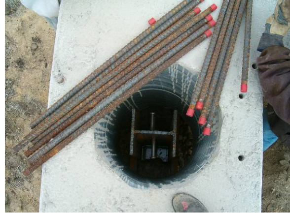
Figure 6. Abutment CMP blackout
