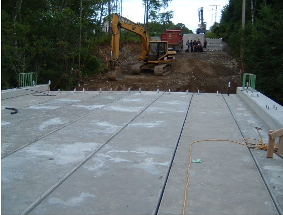
Figure 9. Looking eastbound on the Lamson Bridge Project across the top of the adjacent prestressed voided deck beams. The beams were post-tensioned transversely so the deck would act as a single unit (note the precast segmental retaining wall units on-grade in the background, next to the local residents who took interest in the construction progress).
