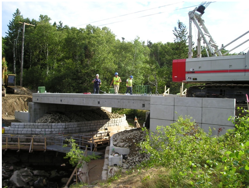
Figure 8. Looking westbound on the Lamson Bridge construction site. Note the precast concrete backwall, the precast, segmental retaining wall panels, and the post-tensioning duct pockets in the fascia beam.
