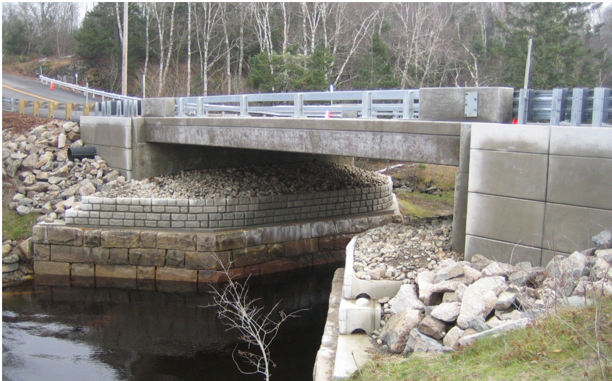
Figure 11. The completed Lamson Bridge Project.
