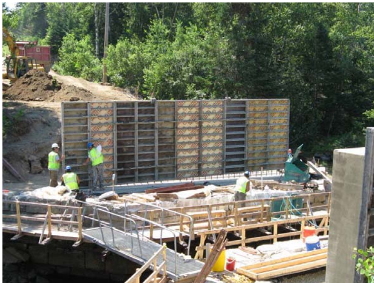
Figure 7. Placement of the abutment forms for the Lamson Bridge.
