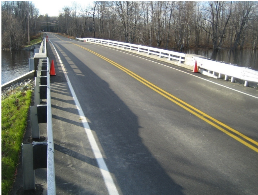
Figure 26. Boom Birch post-construction pavement.
