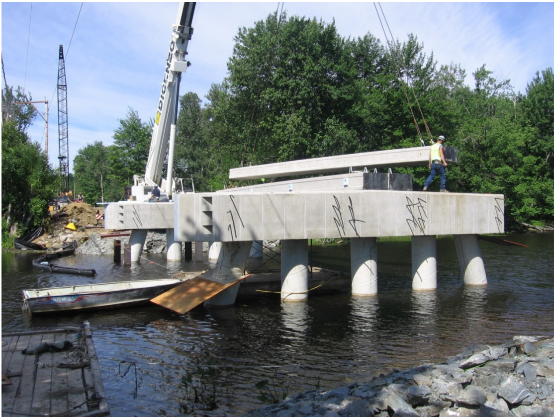
Figure 17. Placement of the superstructure beams.
