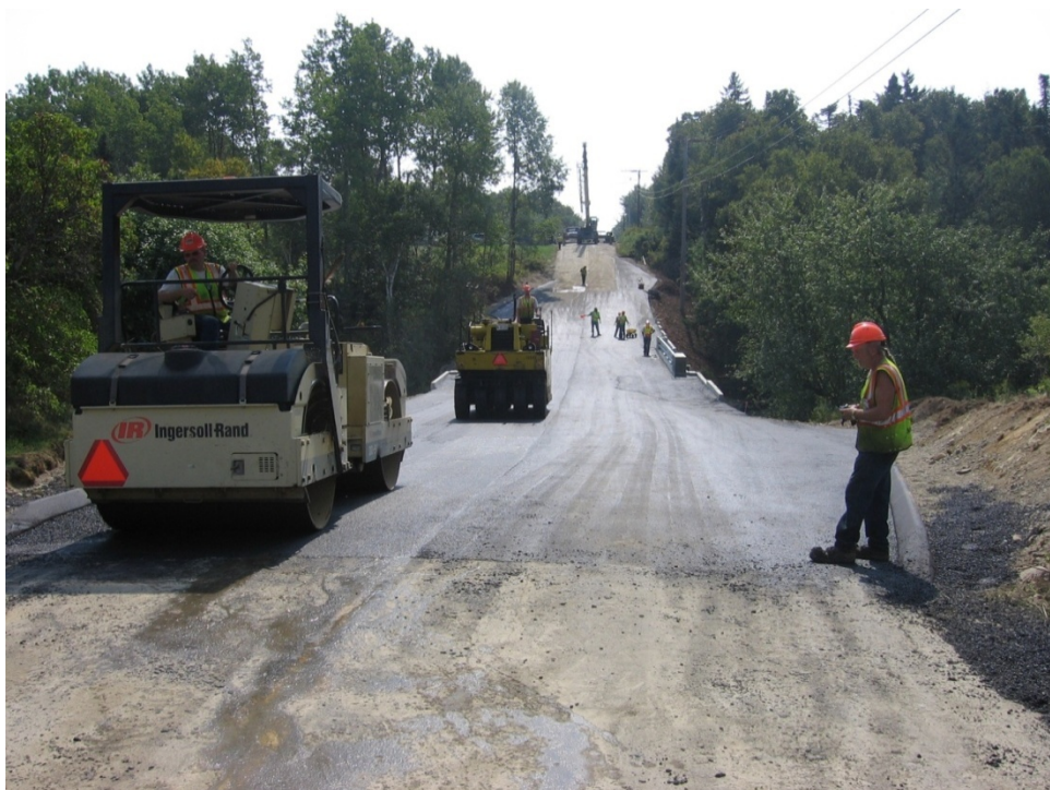
Figure 10. Placing the asphalt concrete wearing surface on the Lamson Bridge.
