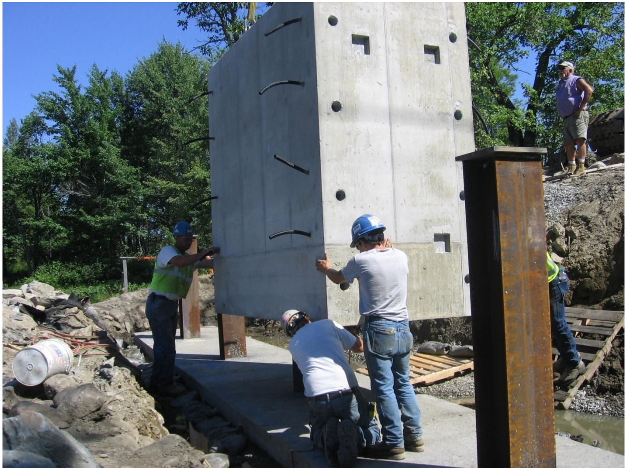
Figure 15. Installation of the precast bridge abutment.
