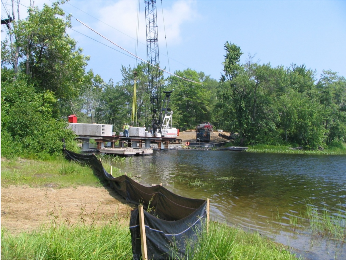
Figure 16. Installation of the precast post-tensioned pier caps.
