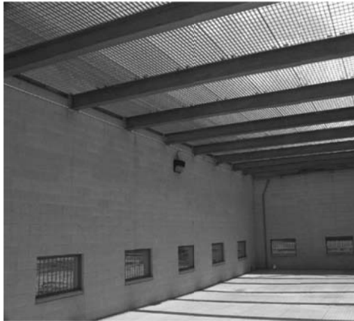
Figure 1.7 Bearing Wall Building Photo courtesy Douglas Steel Fabricating Corporation
