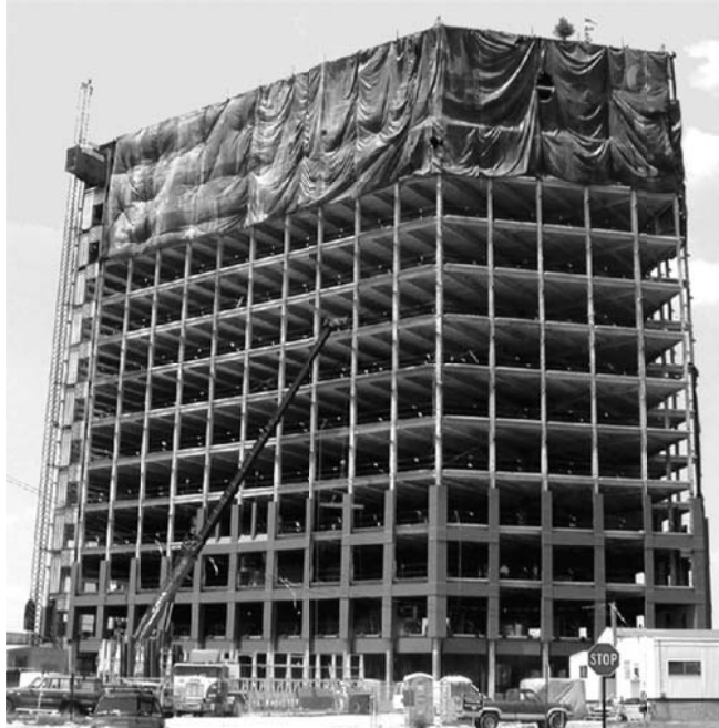
Figure 1.12 High-Rise Building Structure Photo courtesy Douglas Steel Fabricating Corporation
