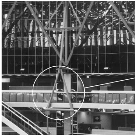
Figure 1.2 Use of Tension Members as Hangers
