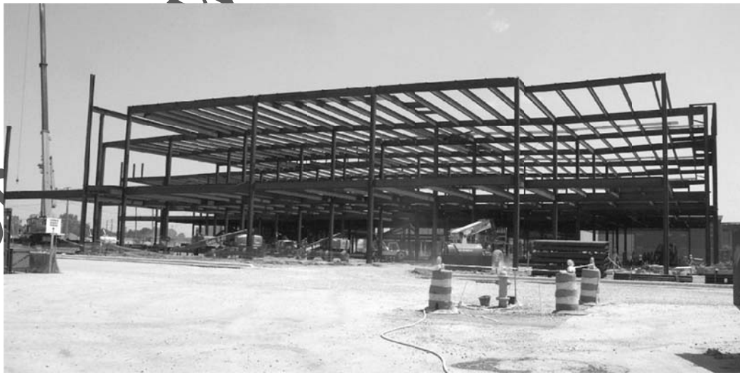
Figure 1.8 Beam-and-Column Building Photo courtesy Douglas Steel Fabricating Corporation
