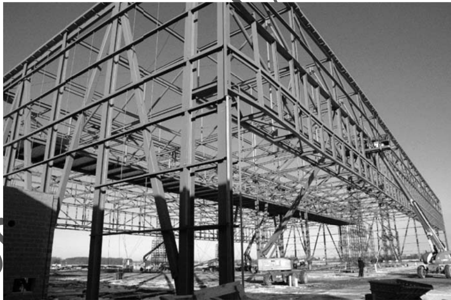
Figure 1.11 Long-Span Structure Photo courtesy Douglas Steel Fabricating Corporation
