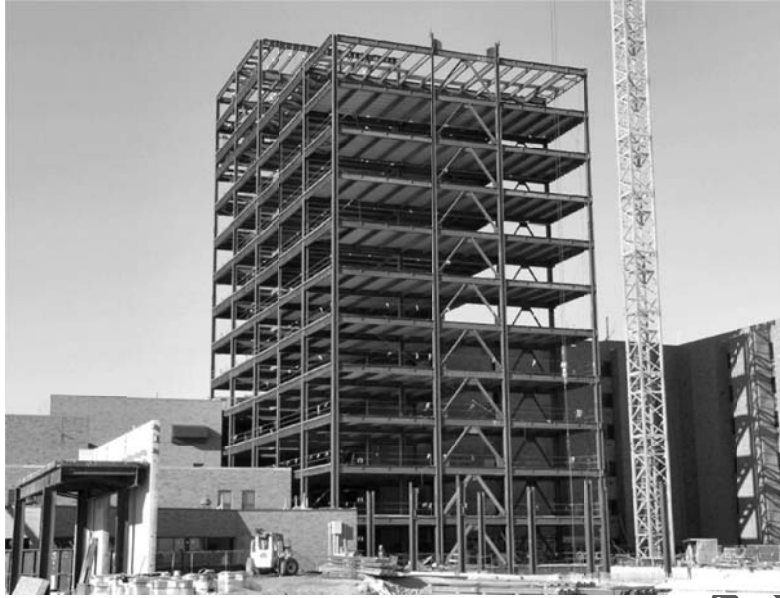
Figure 1.9 Braced Beam-and Column Building Photo courtesy Douglas Steel Fabricating Corporation
