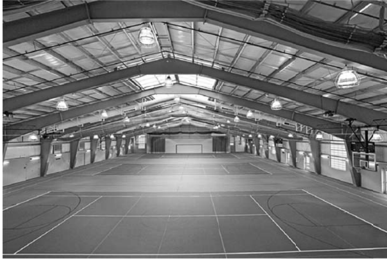
Figure 1.14 Pre-engineered Metal Building Photo courtesy Metal Building Manufacturers Association
