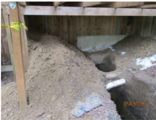
Figure 5. View of work area under deck of house where spoils had been placed at the open edge of the trench
