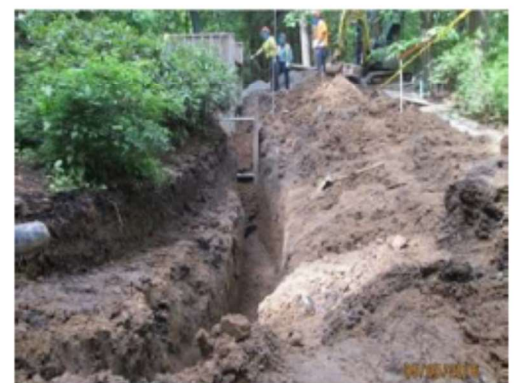
Figure 4. View from house showing trench work area and general soil conditions
