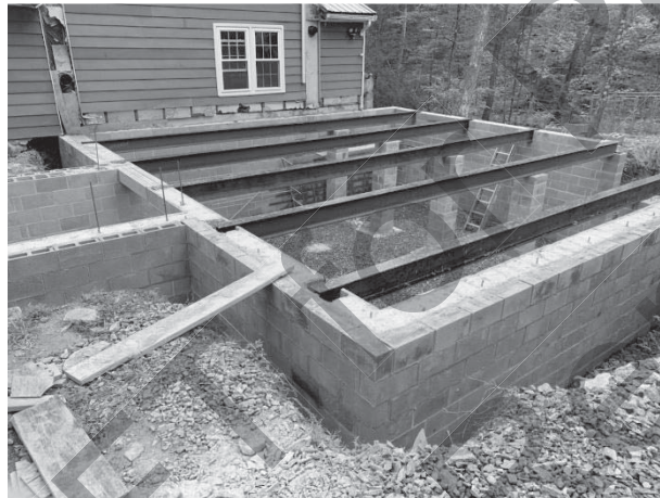
Figure 1.7 Bearing Wall Photo courtesy Providence Engineering
