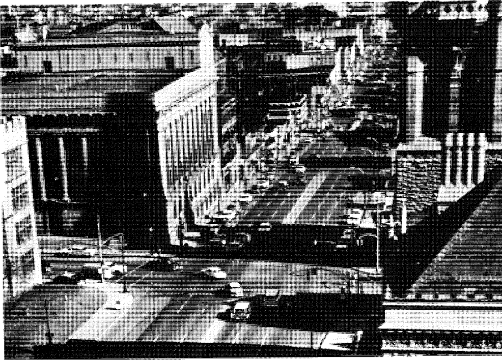
Principal street in central business district providing six traffic lanes and two parking lanes. Note traffic making left-turn maneuver in foreground on advance signal control before opposing traffic starts.
