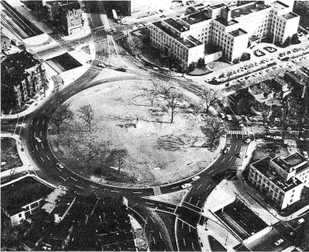
Rotary intersection in urban area. Grade separation used to carry major traffic flow underneath. Traffic signals, pavement markings, and raised islands extensively employed to facilitate traffic movement.
