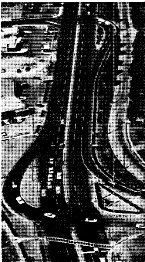
Special signalized "jug-handle" turning lanes minimize intersectional friction on this suburban arterial street. Note frontage road on right minimizing land use interference and conflicts from land use on left.
