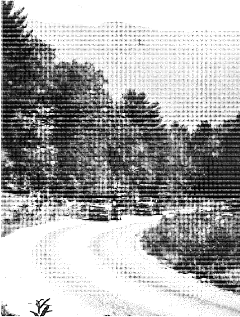
Winding 2-lane rural road with steep grades and carrying significant truck volume has greatly restricted capacity.
