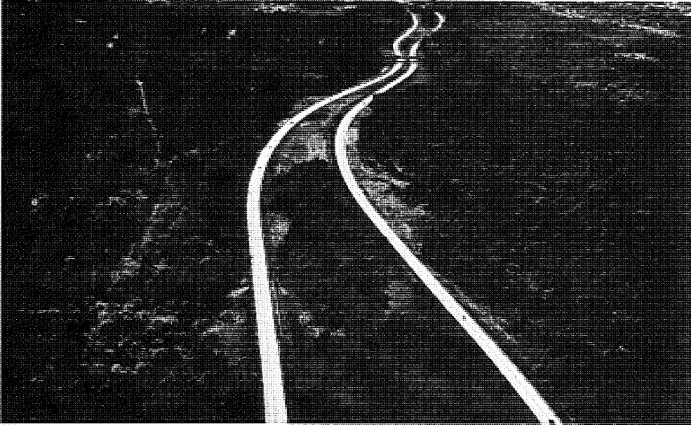
Multilane freeway retains high capacity level by few changes in alinement and by grade reduction. Note variable median width in adverse terrain.
