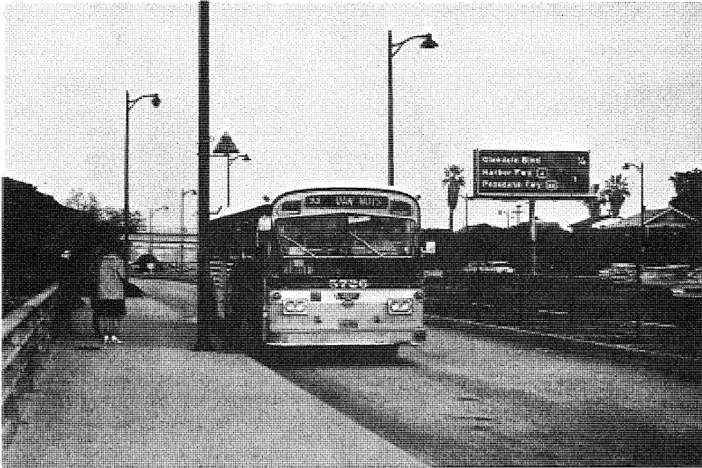
Exclusive bus loading area adjacent to a freeway. Note fencing for passenger protection.
