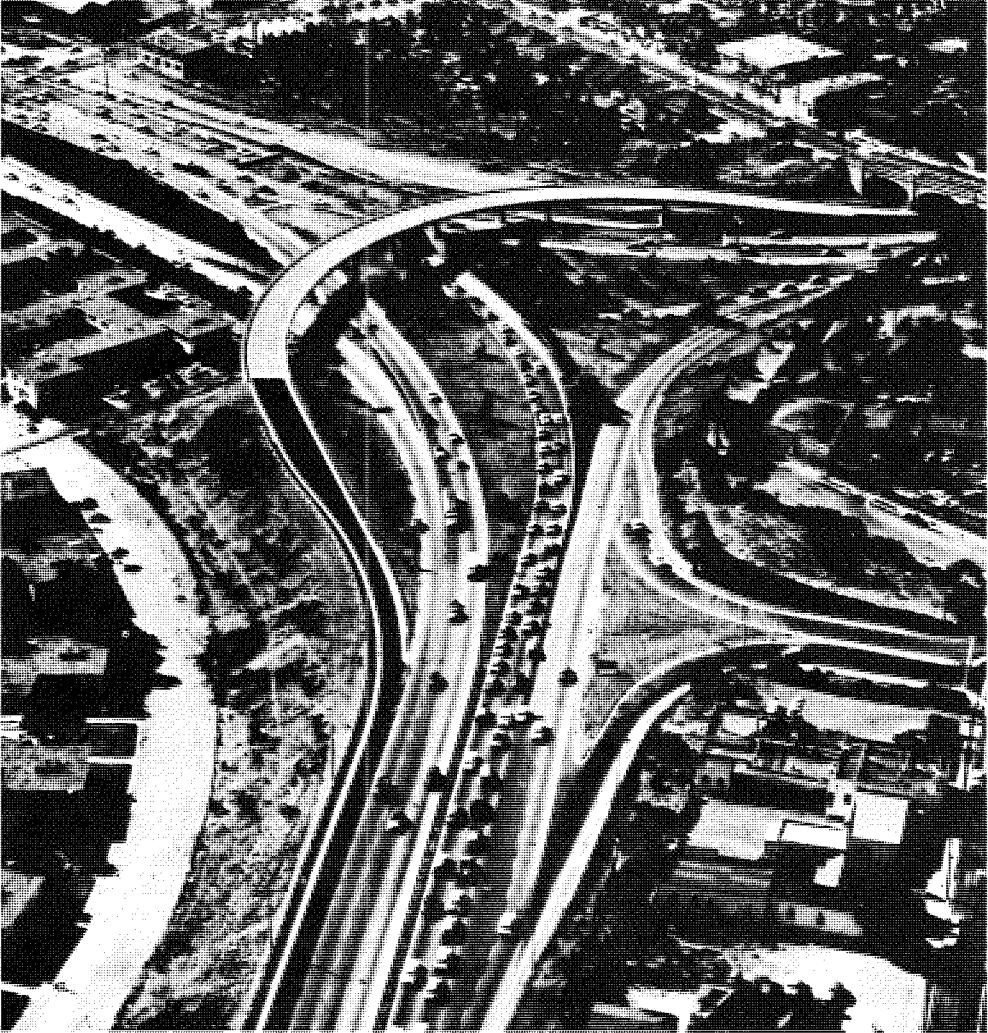
Unbalanced traffic flow. Predominant flow is from bottom to top of photo; counter movement is relatively light. Note direct left-turn connection from highway at right and channelization used to separate ramps at right center.
