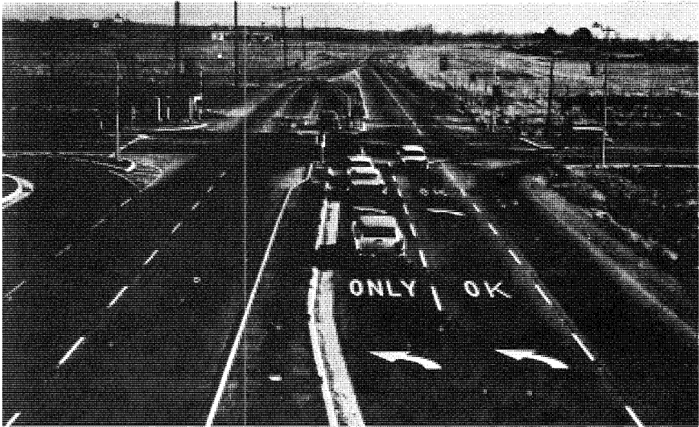
Separate left-turn lane at high-capacity rural signalized intersection. Note right-turn lane from cross road at extreme left.
