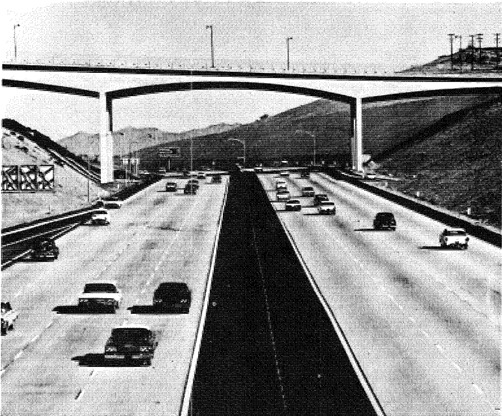
Grade separation over 8-lane freeway. Paved median provided with edge striping for visibility and fence in center. Note provision of shoulders and adequate side clearances at structure.
