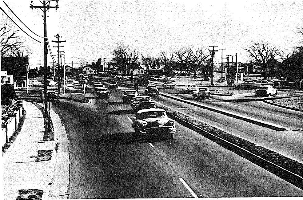
Traffic interruptions from roadside development and intersections on this divided highway without control of access restrict service volumes.
