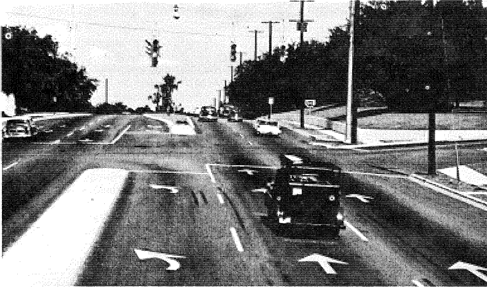
Separate left-turn signal indications and exclusive left-turn lanes at intersection on major urban divided highway.
