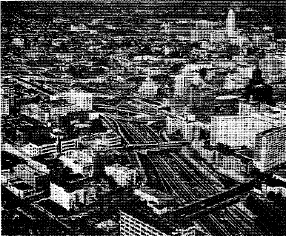
Urban freeway adjacent to central business district. Grade separations carry city streets over this high-volume full-control-of-access facility.
