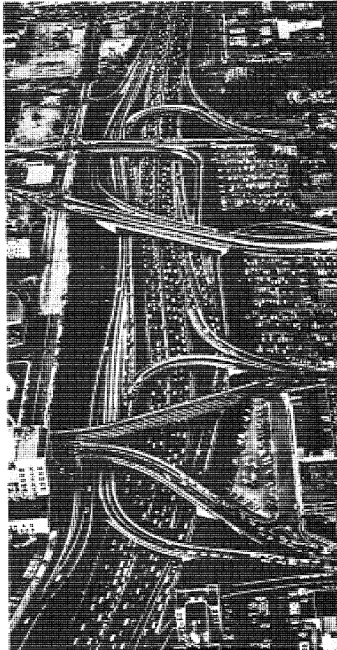
Downtown area freeway, showing ramps to and from cross streets.
