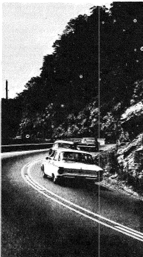
Lack of auxiliary climbing lane, adequate shoulders, and proper alignment reduce capacity of this 2-lane highway.
