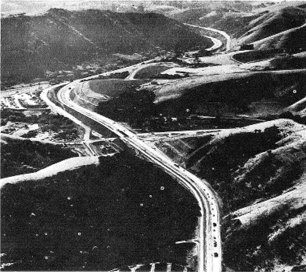
Proper fitting of this 4-lane highway into difficult terrain reduced severe alignment effects that could greatly reduce capacity.
