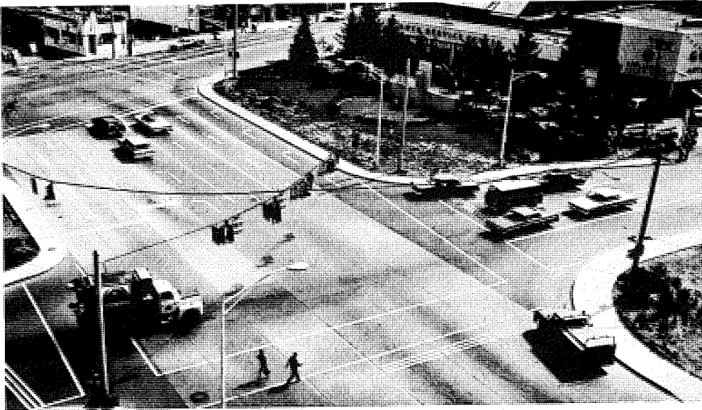
Well-marked pavement and prohibition of parking expedite traffic at this pair of intersections in an outlying business area.
