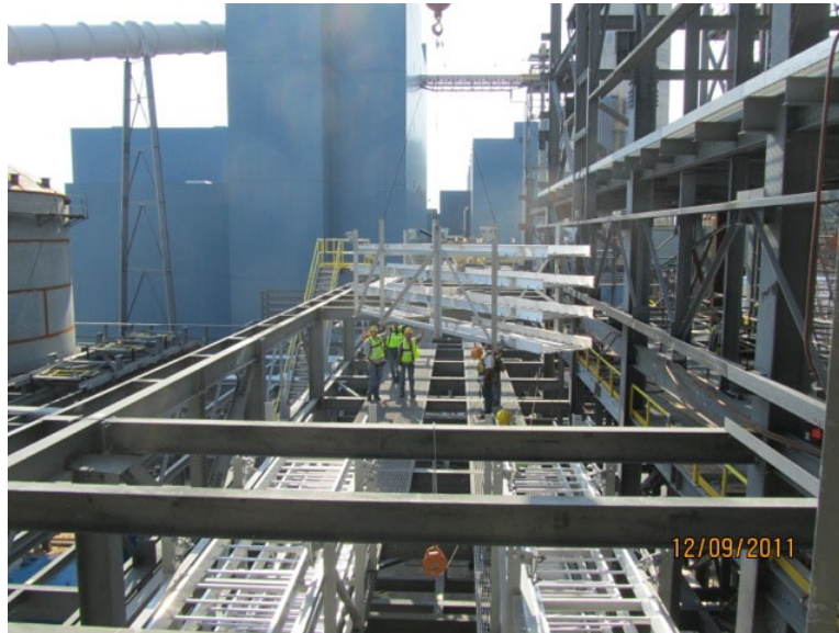
Figure A12.10: Cable tray being lifted into place (Picture provided by URS Corp.)
