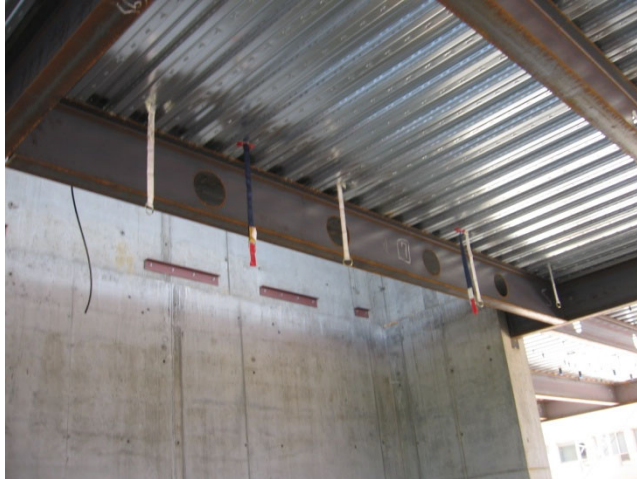
Figure A12.5: Concrete straps attached to slab reinforcement above
