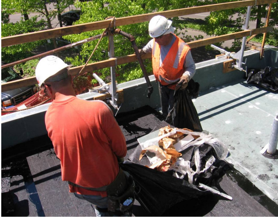
Figure A12.9: Construction workers placing insulation on the roof (Rajendran and Gambatese 2013)
