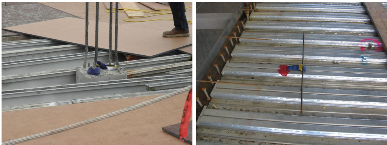
Figure A12.3: Concrete strap attached to column reinforcement (left), and floor reinforcement (right)
