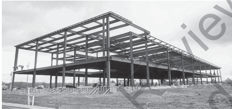
Figure 5.1 Columns in a Multistory Building Photo courtesy of Greg Grieco
