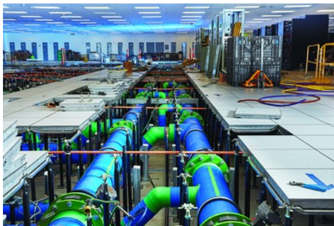
In preparation for El Capitan, upgrades to Livermore's primary machine room included scaled-up, energy-efficient cooling infrastructure. Water flows through the green and blue pipes without the use of chillers.
