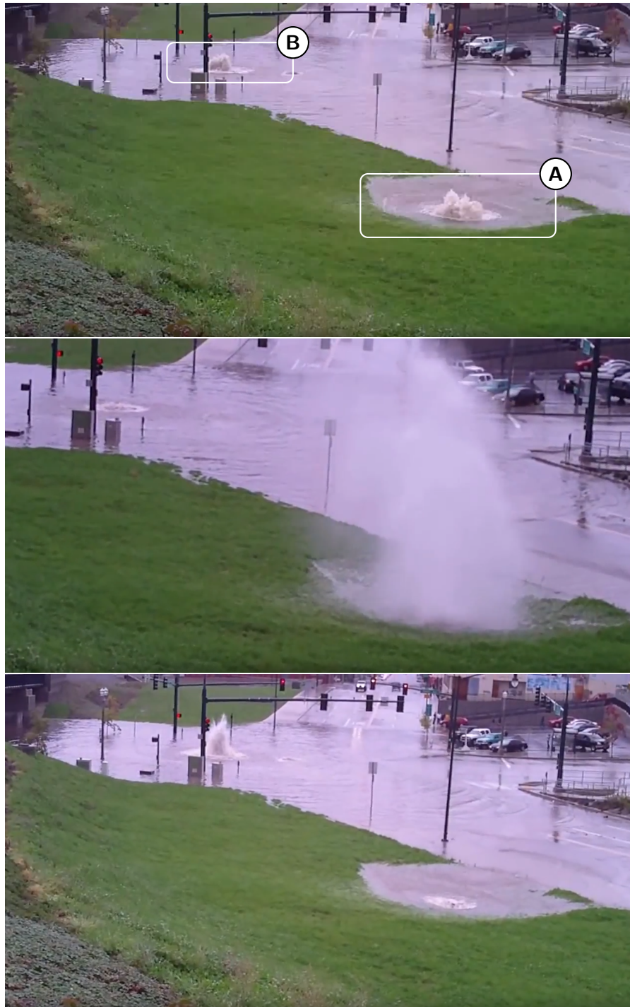
Figure 1.7: Sewer geyser observed at the intersection of Pacific Ave and S Tacoma Way, Tacoma, WA (screenflot, 2013).
