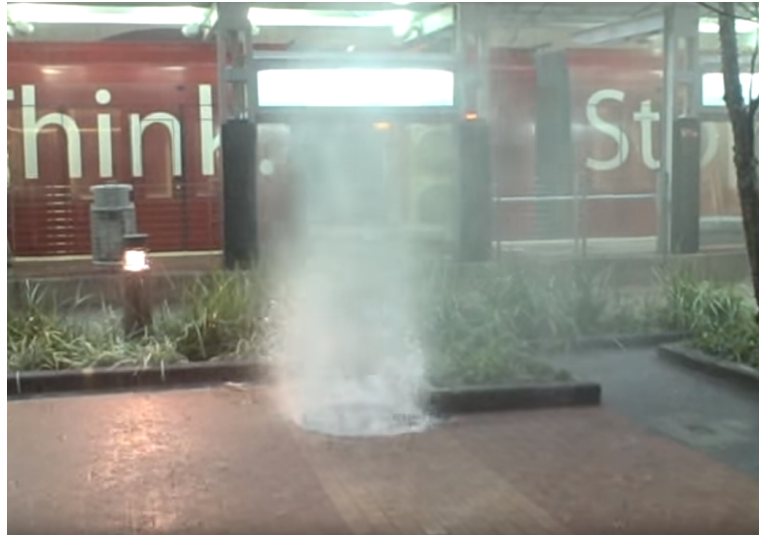
Figure 1.6: An example of ejecting air-water mixture overflow observed in downtown Houston, TX (NYCYankinTexas, 2012).
