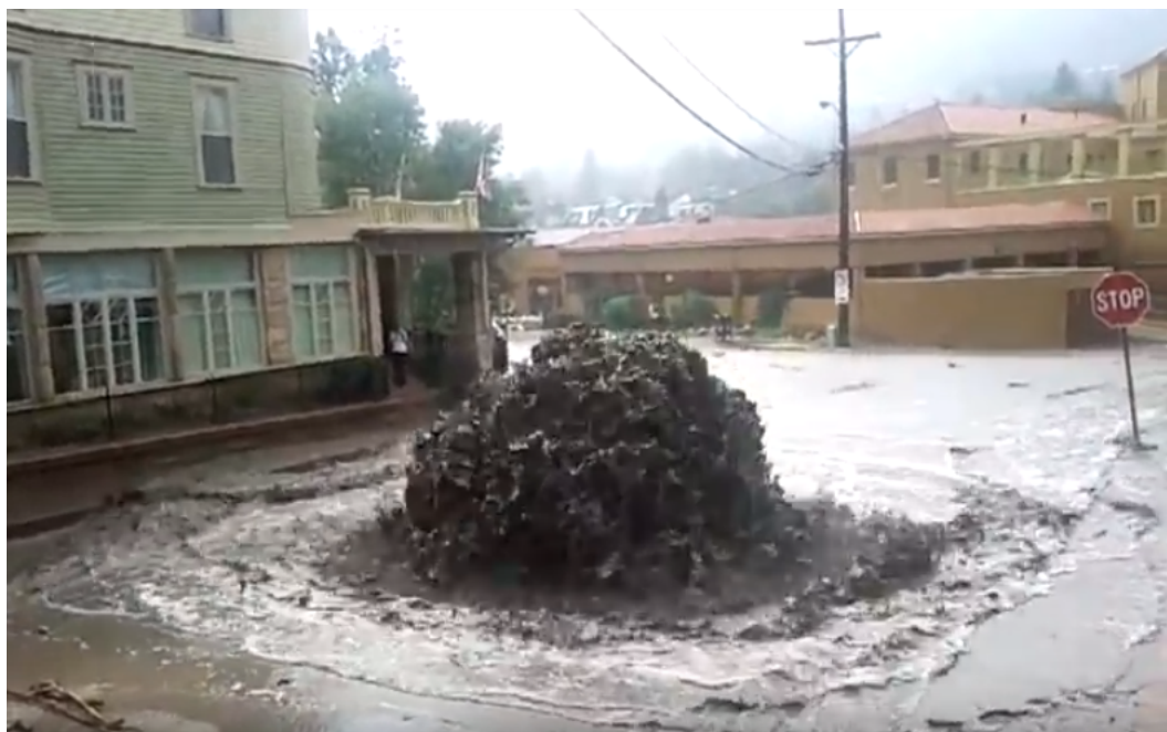
Figure 1.5: An example of liquid volume displacement sewer overflow from the Canon Ave storm sewer system (JS4IV, 2013).
