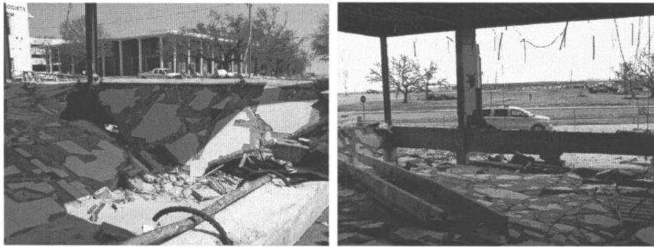
**Fig. 23.** Liquefaction-induced scour under fill-supported first-floor slab
