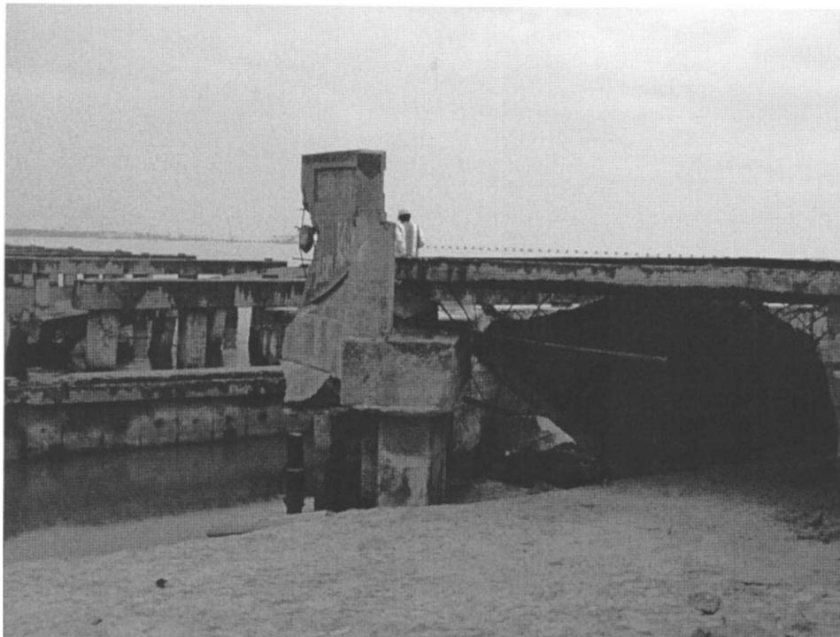
**Fig. 25.** Up to 4.5 m (15 ft) of scour around abutment exposing piles below abutment
