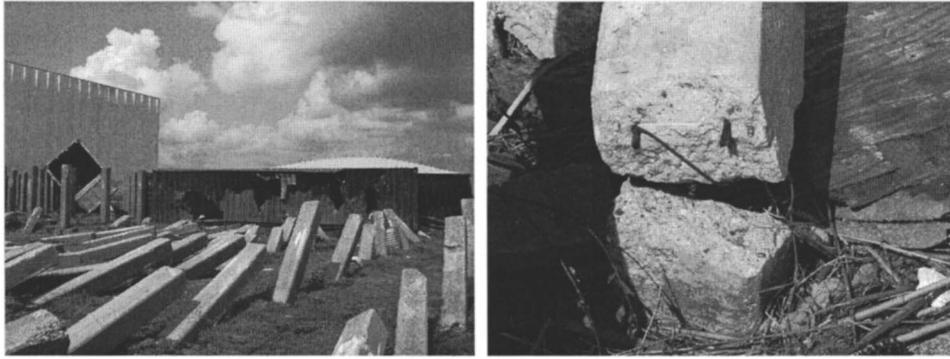
**Fig. 30.** Bending failure of piles due to shipping container impact and damming effect
