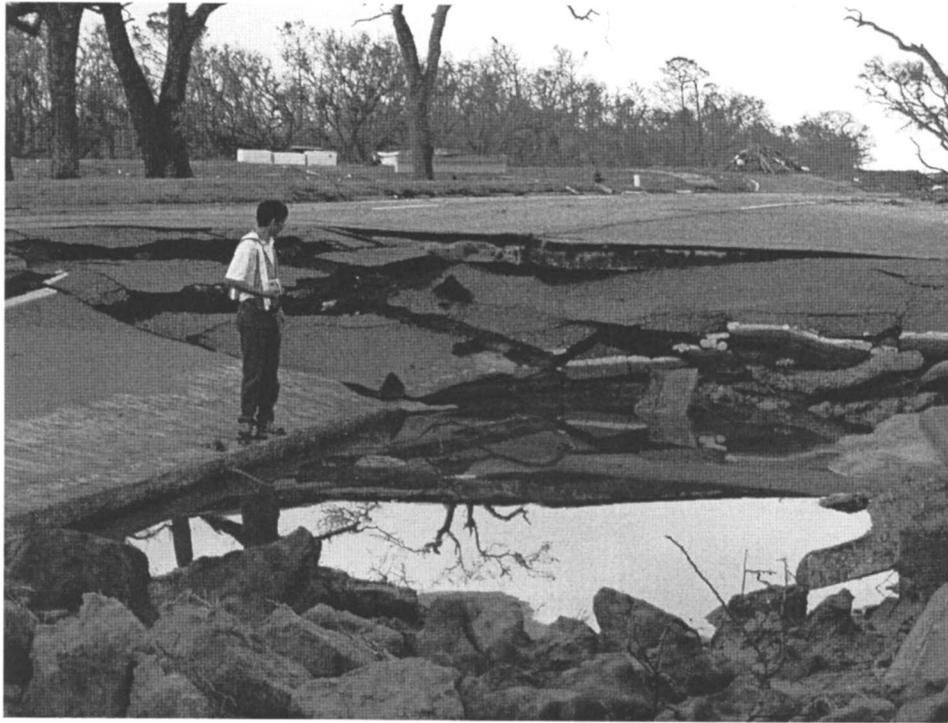
**Fig. 24.** Sinkhole-like crater left by scour of liquefied subgrade below coastal highway
