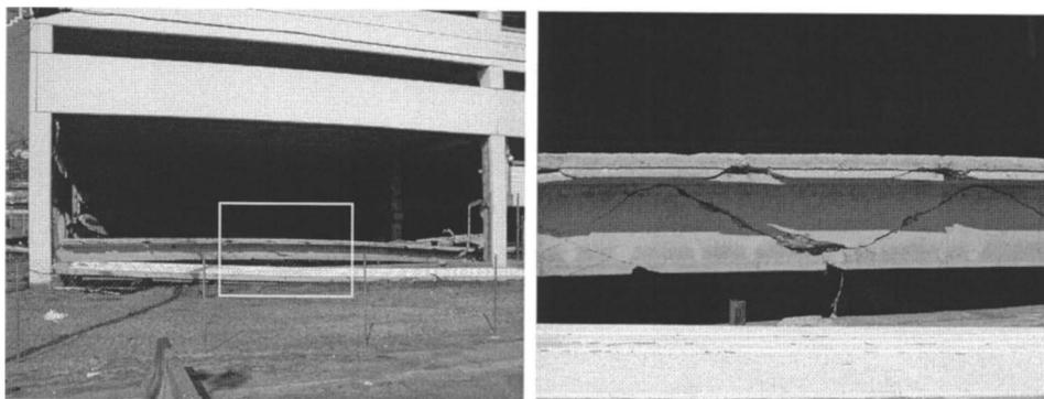
**Fig. 11.** Double-tee negative bending failure—parking structure in Biloxi
