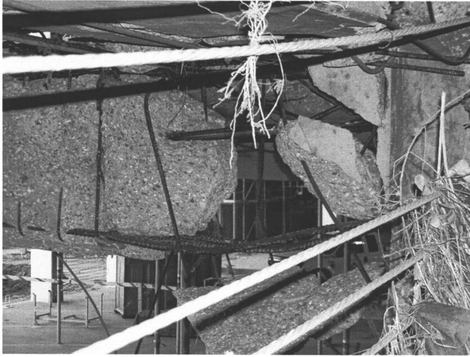
**Fig. 15.** Shear failure of posttensioned beam supporting one-way posttensioned slab
