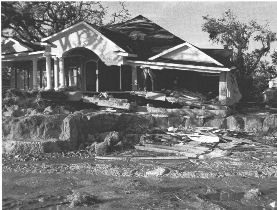
**Fig. 27.** Scour under foundations leading to partial collapse of residence
