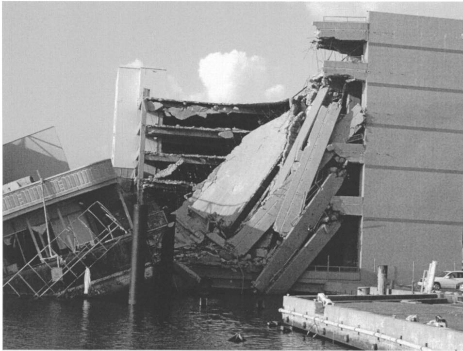
**Fig. 19.** Progressive collapse of parking structure due to barge impact damage to lower-level columns
