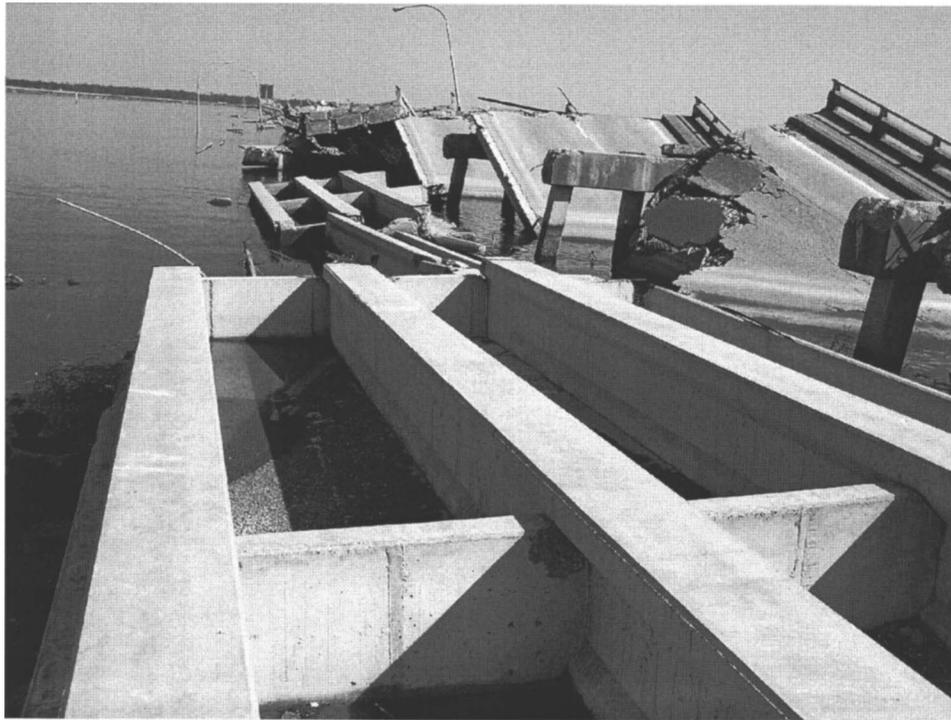
**Fig. 3.** Girders, bridging, and bulkheads potentially trap air below deck of US 90 highway bridge over Biloxi Bay
