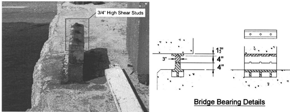
**Fig. 8.** Rocker bearing details at US 90 highway bridge over Bay St. Louis (1 in.=25.4 mm)
