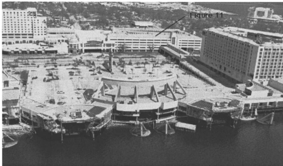
**Fig. 2.** Grand Casino, Biloxi, with inland parking garage that suffered collapse of the second-level double-tee floor system (Fig. 11) (Photo courtesy of U.S. National Oceanic and Atmospheric Administration/Department of Commerce)
