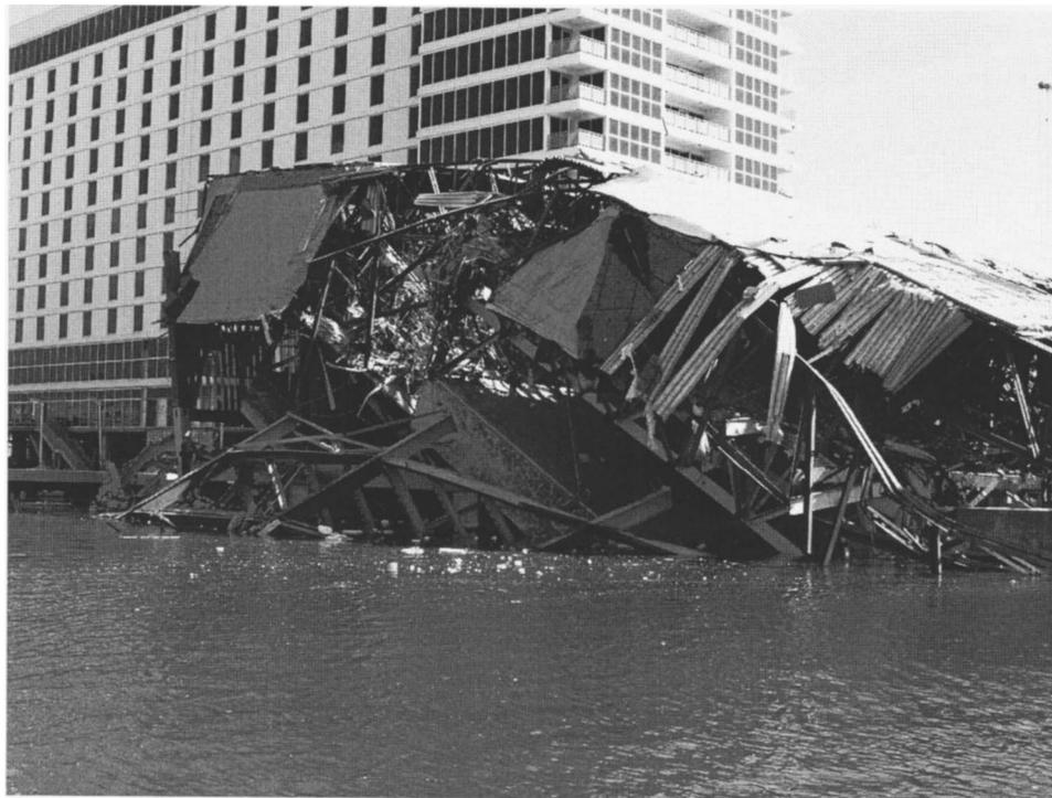
**Fig. 18.** Hard Rock Casino barges enclosed by fixed exterior steel structure
