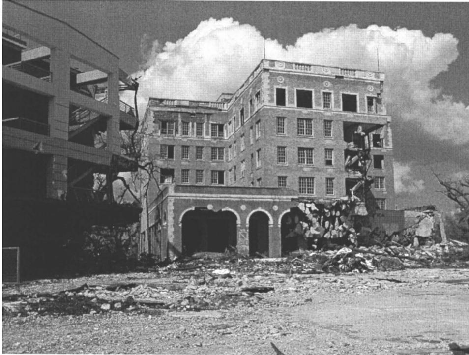
**Fig. 21.** Damage to cast-in-place reinforced concrete building caused by impact of adjacent barge
