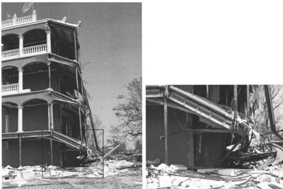
**Fig. 29.** Shipping container damage to steel pipe columns supporting balconies
